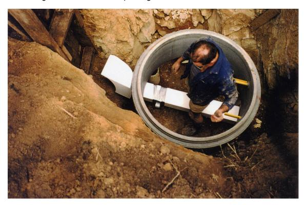
The core end is placed into the side branch.
