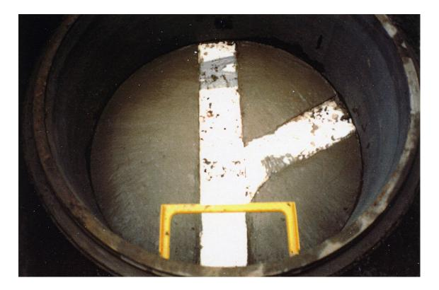
After the concrete has cured, the poly-formers are removed leaving the finished channel, as shown below.
