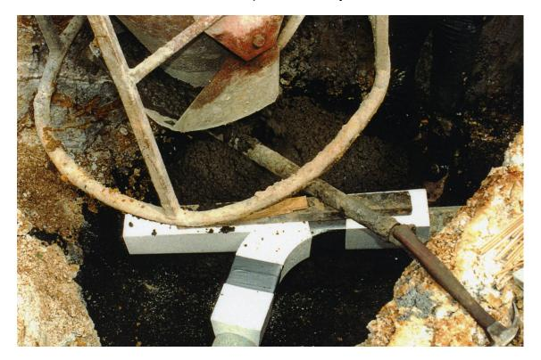
Concrete is poured into the outlet region as shown, then into the final segment of the manhole base.
